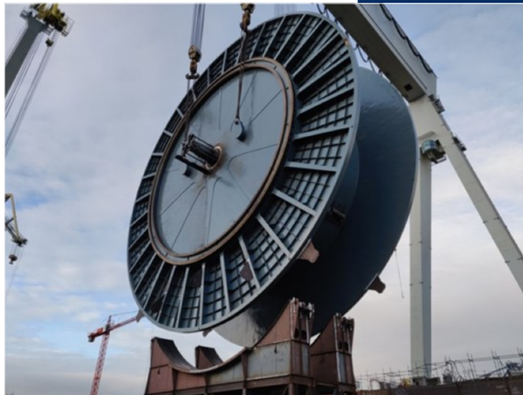
SS7 -R Diameter – 32 m, Total Width – 15 m, Total mass – 820 ton
